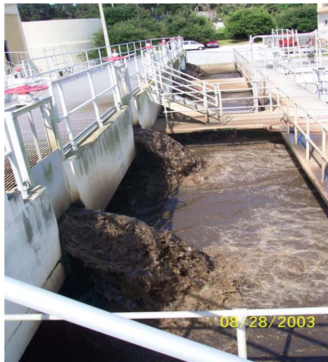
Figure 2 – Picture showing the MLR flow input into the first anoxic basins at the MSAPCF.
