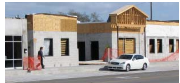
Façade improvement on Cleveland Street
