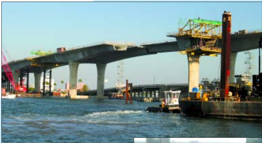
View of Memorial Causeway Bridge taken from mainland facing west.
