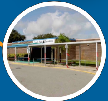
Sandy Lane Elementary School
