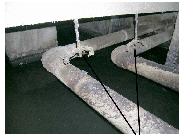
PHOTO 1 REMOVE EXIST. PIPE HANGERS, INSTALL NEW HANGERS. SEE DETAILS SHEET SD-M-01
