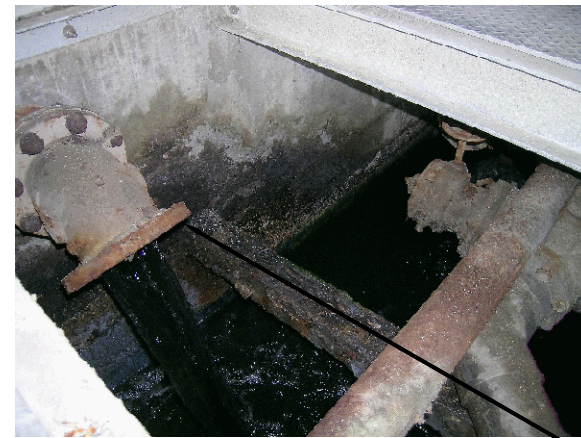
PHOTO 3 EXIST. THICKENER DISCHARGE TO INFLUENT CHANNEL - TO REMAIN IN OPERATION
