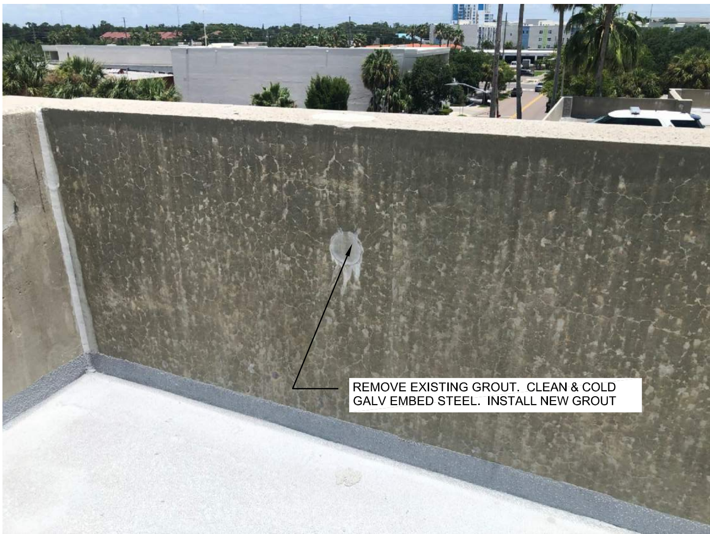
7.5 WALL REPAIR-GROUT POCKET
