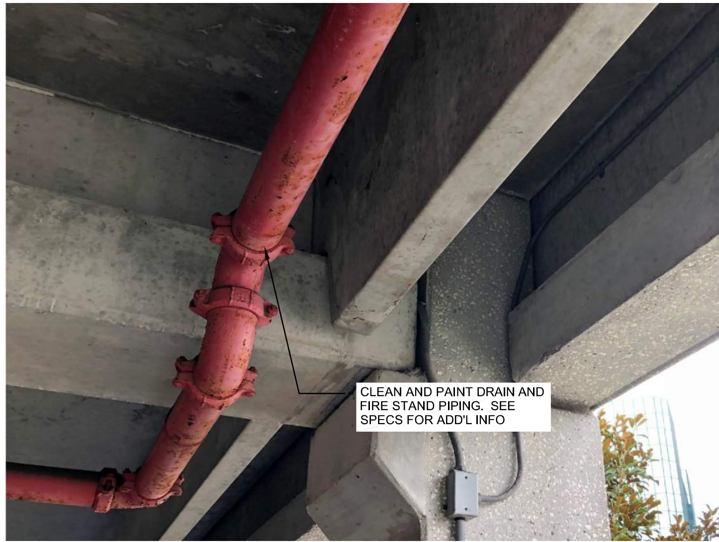
PAINT DRAIN AND FIRE STAND PIPING
