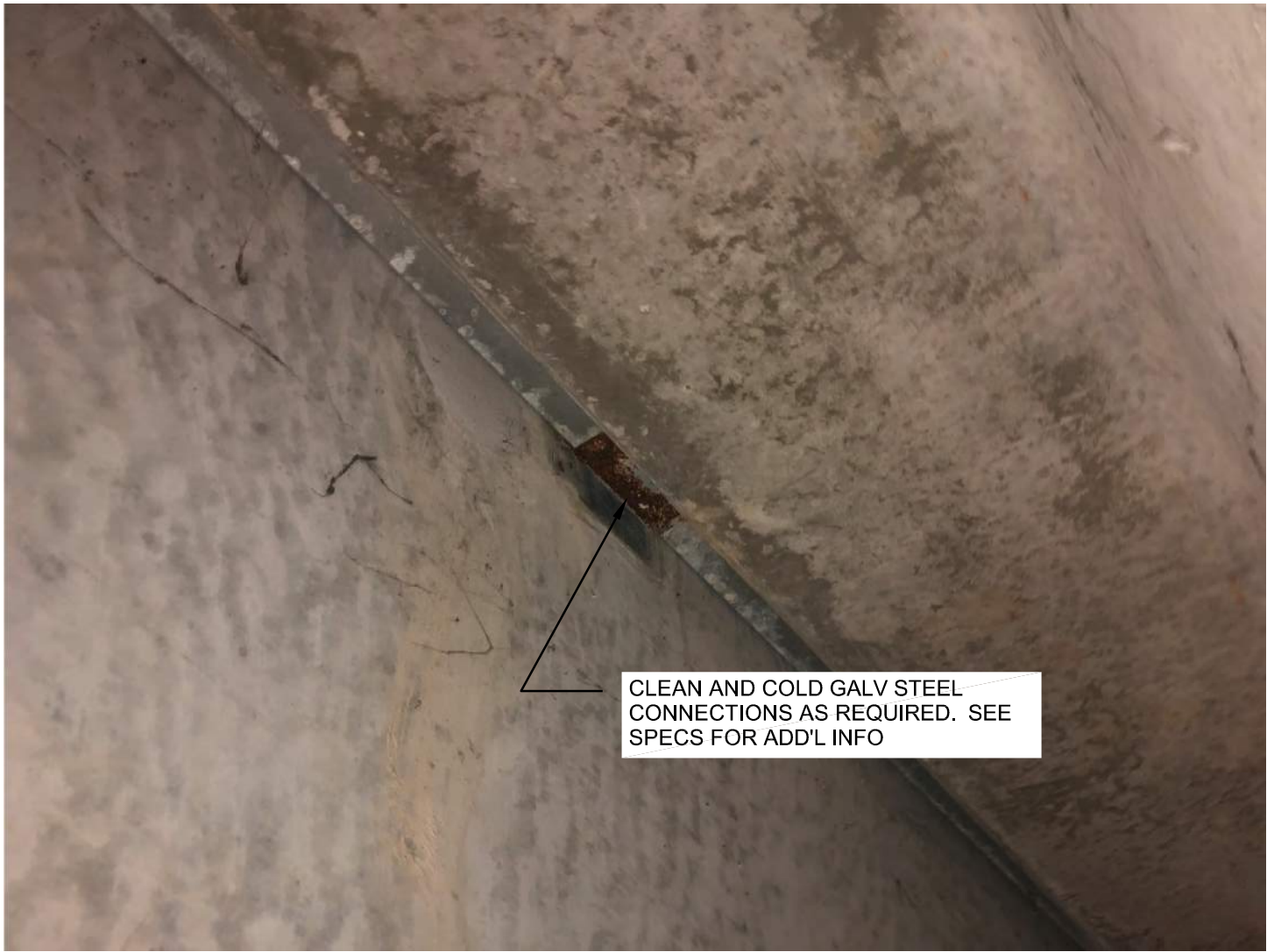
CLEAN AND COLD GALVANIZE STEEL CONNECTIONS
