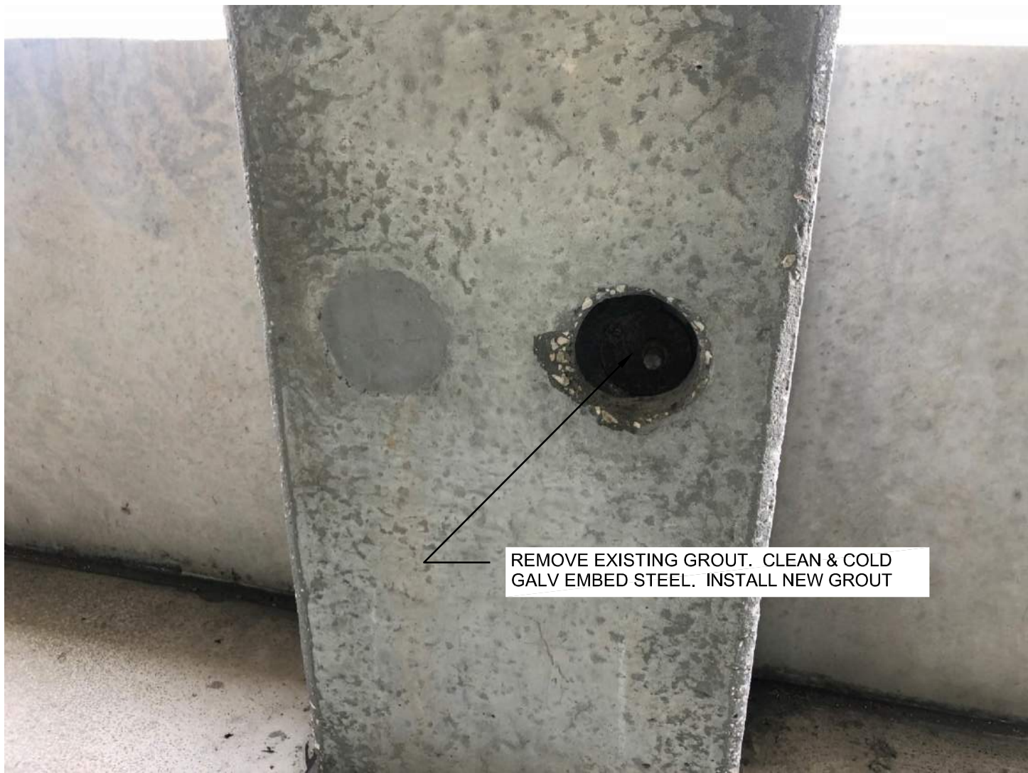
6.5 COLUMN REPAIR-GROUT POCKET
