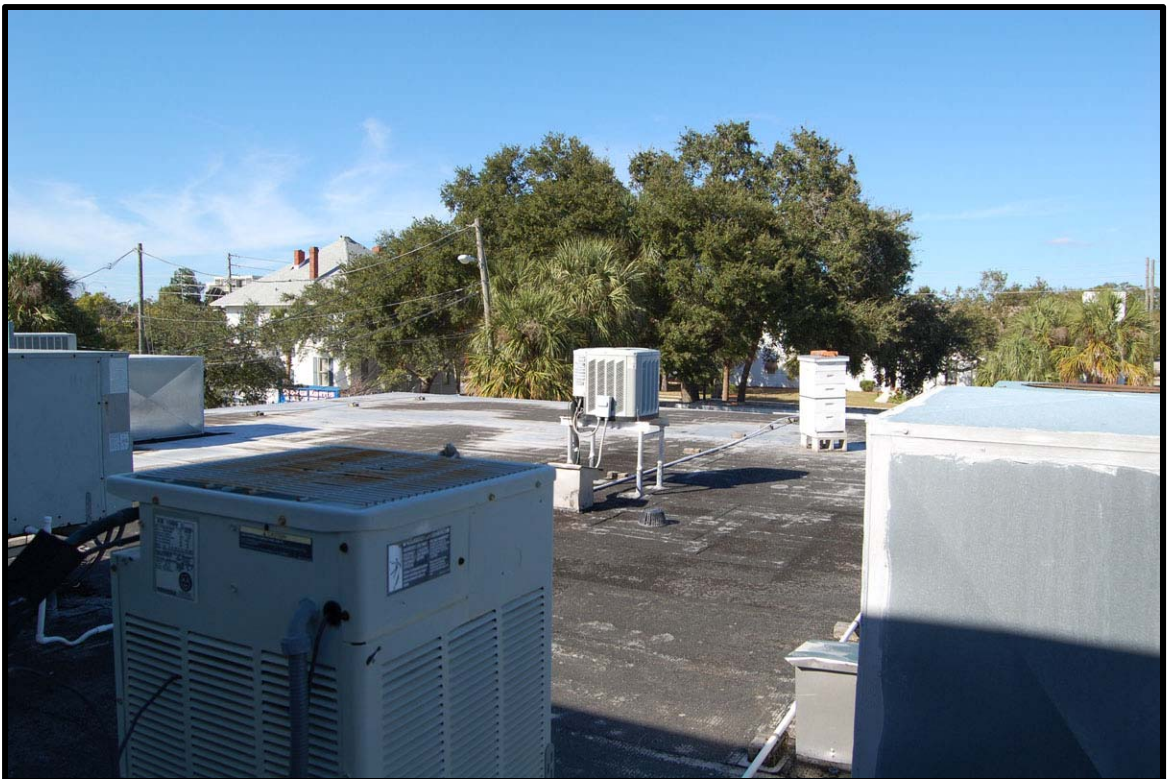
ROOFTOP HVAC UNITS IN REAR SECTION OF BUILDING
