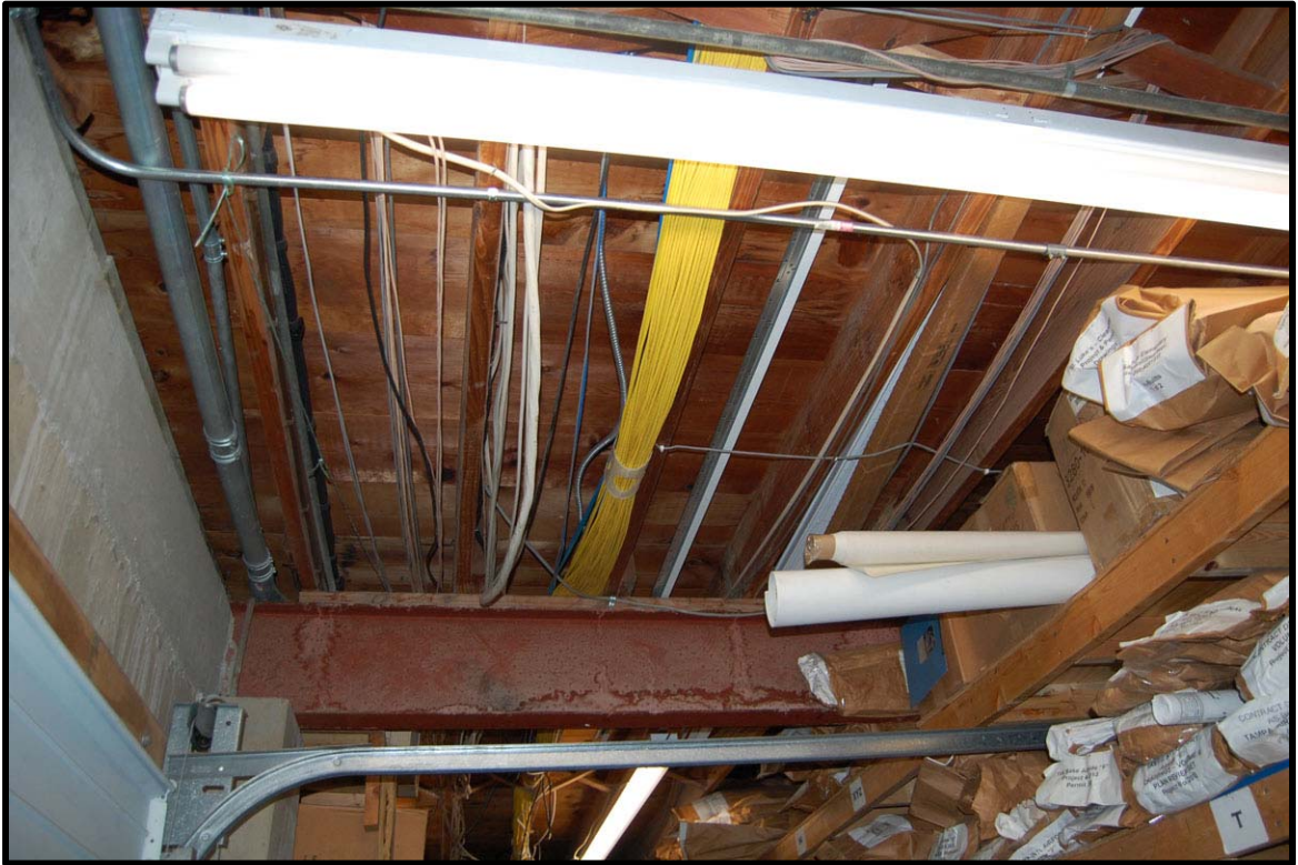
STEEL GIRDER SUPPORTING UPPER STORY WOOD FLOOR JOISTS
