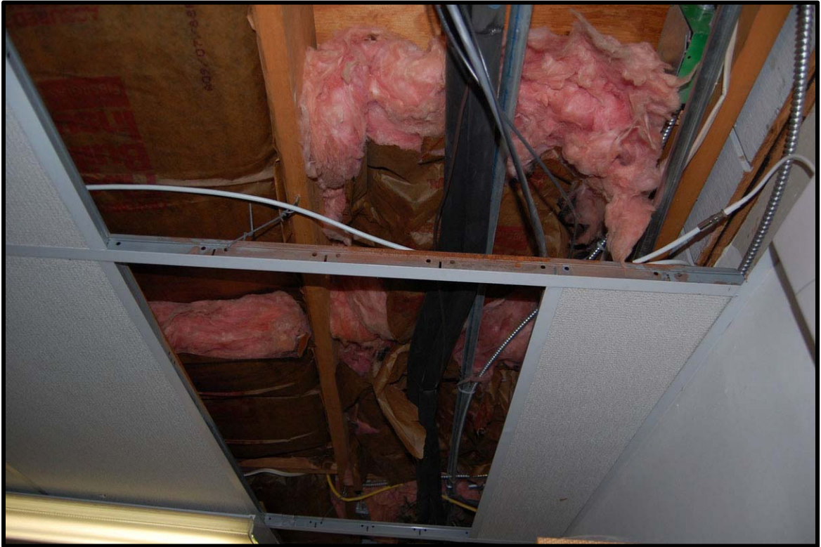
WOOD FRAME ROOF STRUCTURE ABOVE CEILING IN 2 ND FLOOR
