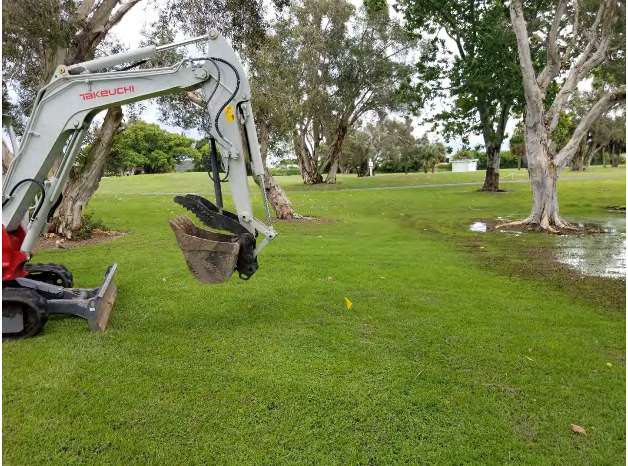
Test Pit TP-42
