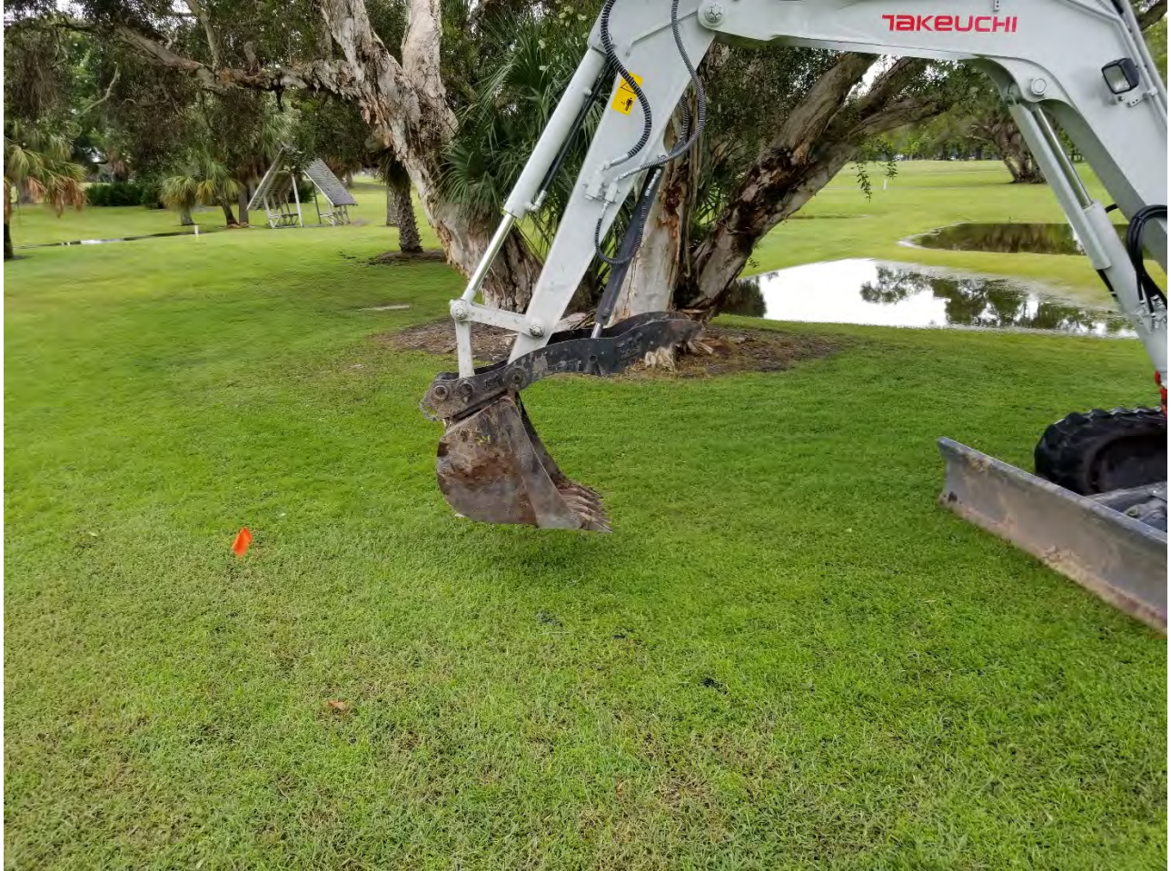
Test Pit TP-30
