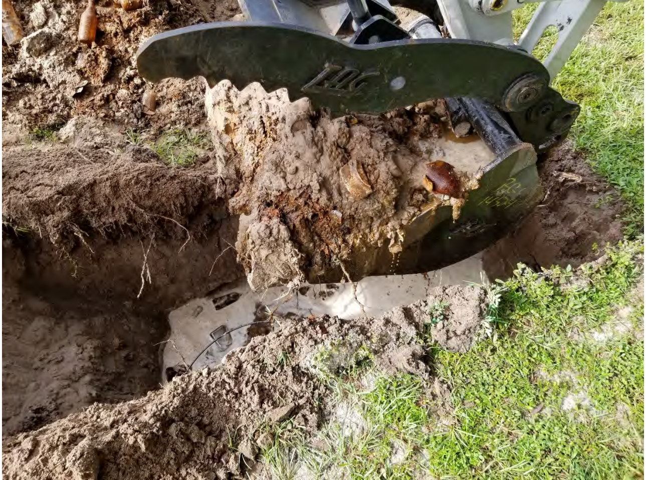
Test Pit TP-37
