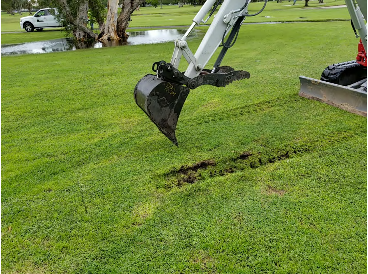
Test Pit TP-45
