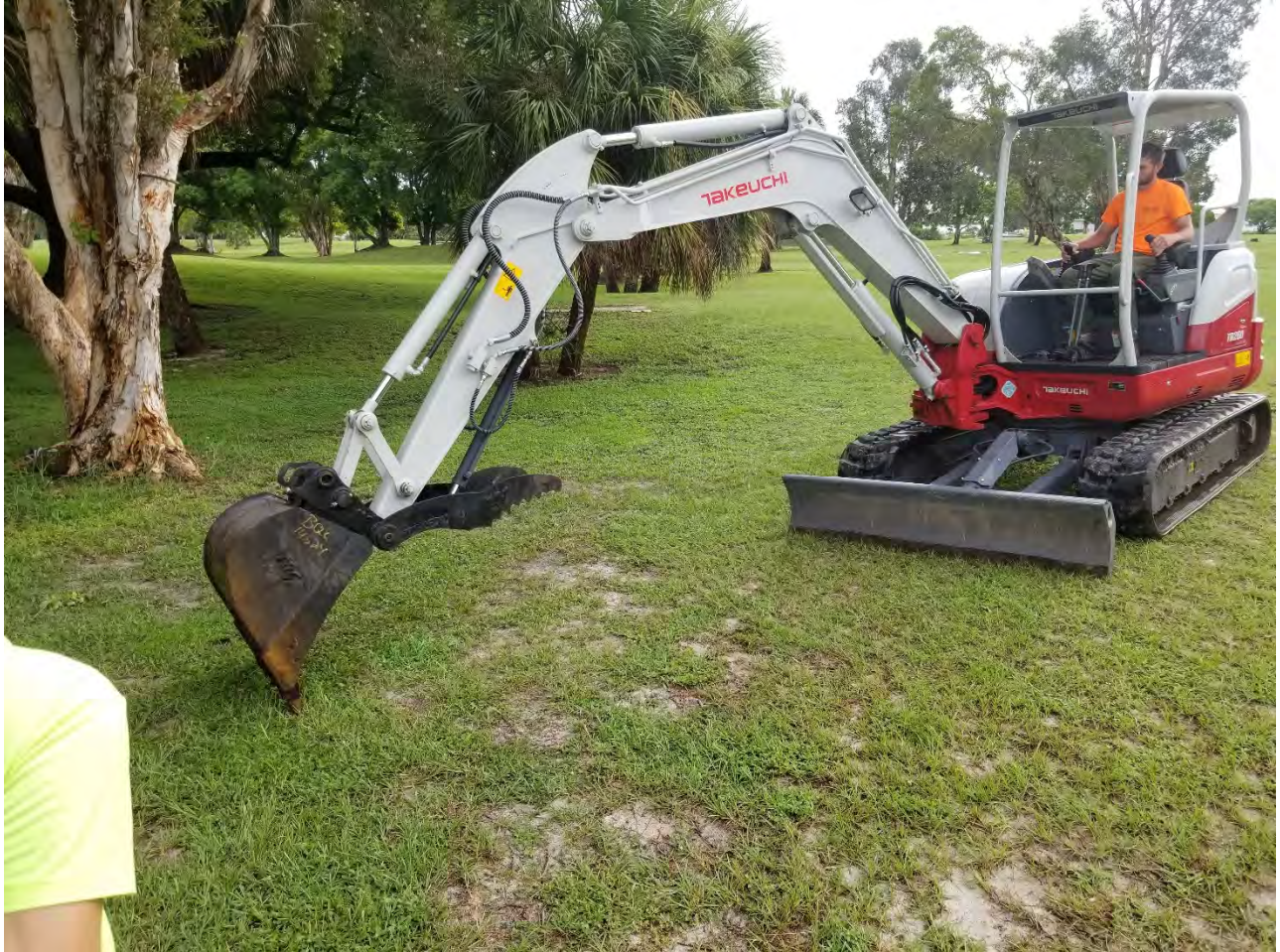
Test Pit TP-37
