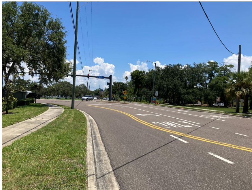
LAKEVIEW ROAD STREET SCENE LOOKING EAST TOWARD SUBJECT ON RIGHT
