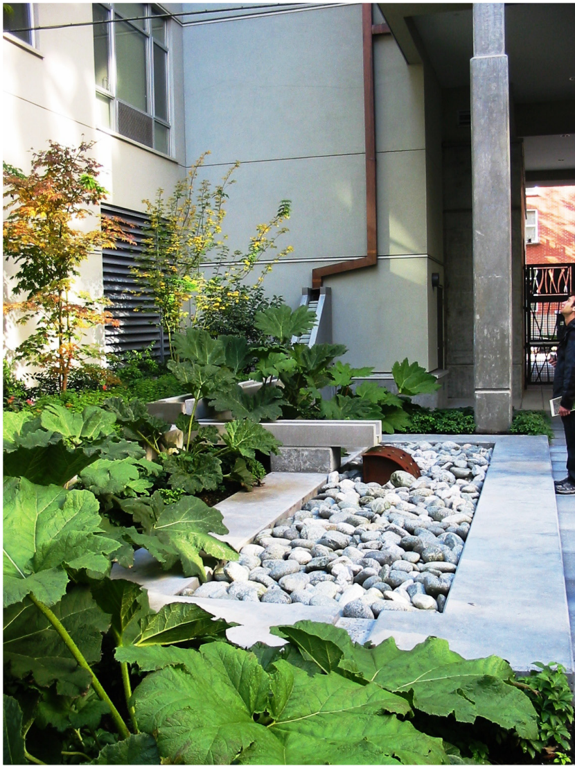
Photo of rain garden capturing roof runoff on Portland, Oregon.
