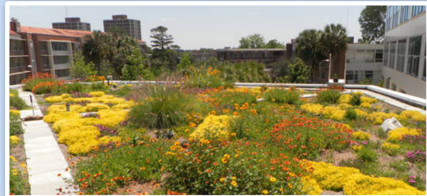
Green roof photos from University of Florida’s Charles R. Perry Construction Yard.
