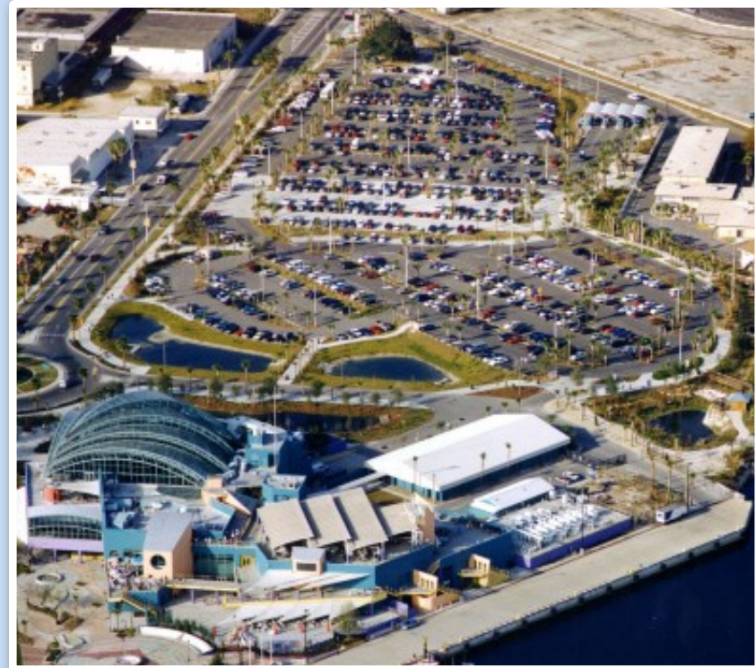
Pervious pavements and vegetated swales at the Florida Aquarium.
