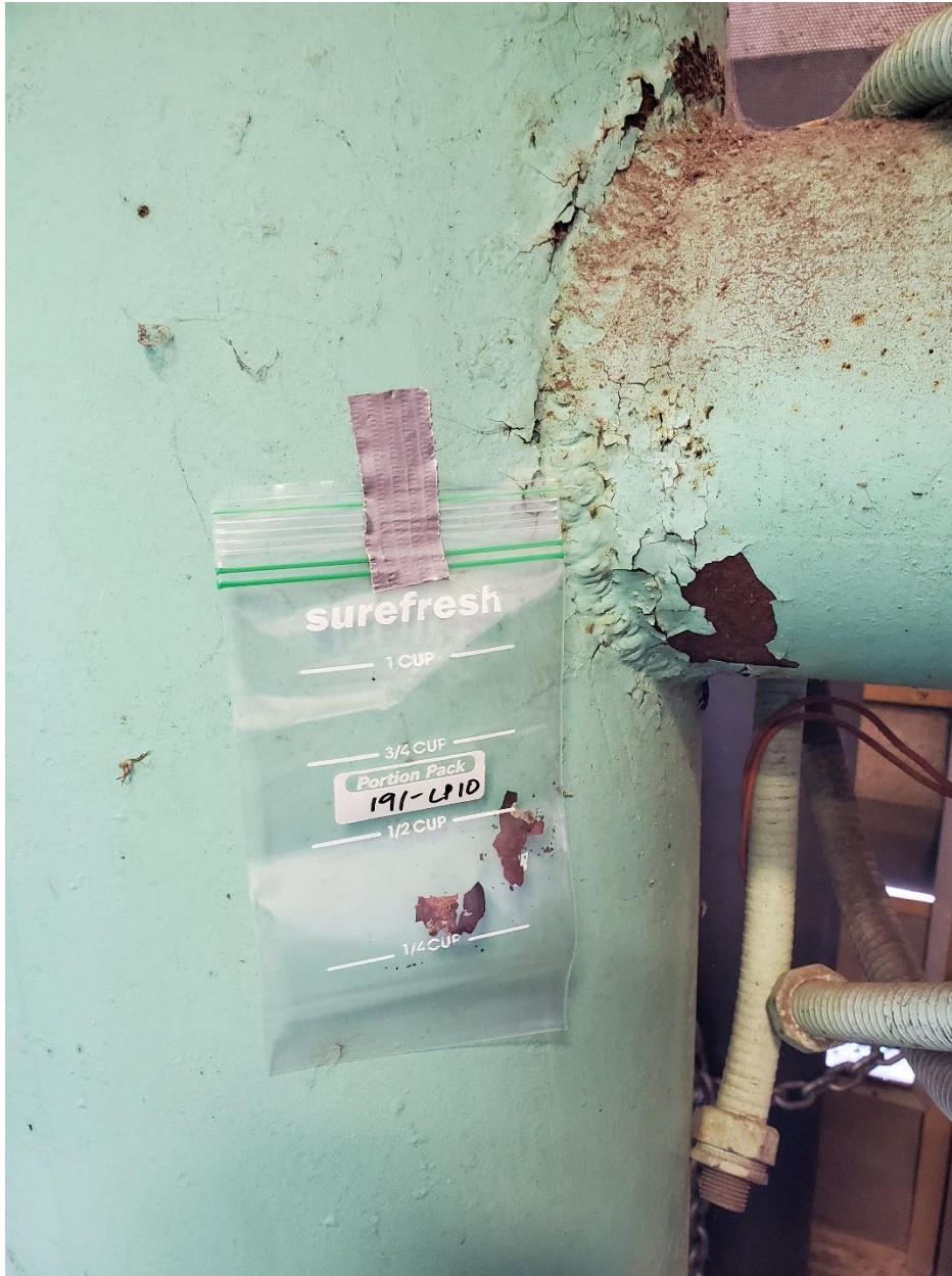
191-LP10: Green Pipe/Crane Paint [NLD]
