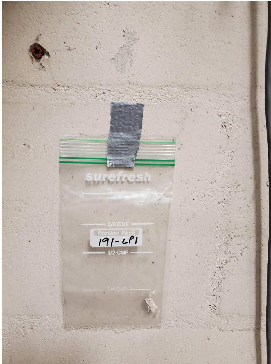
191-LP1: Tan Wall Paint on Concrete Block [NLD]
